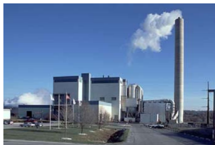
The Montgeny County Plant produces 36 megawatts/hour from 1200 tons/day of waste.
